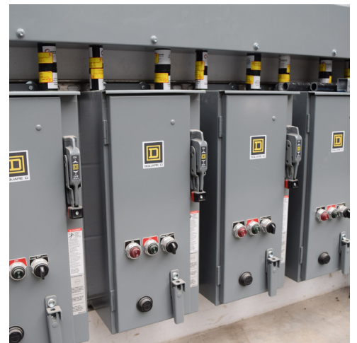
Install Infrastructure Needed for these Upgrades and More
