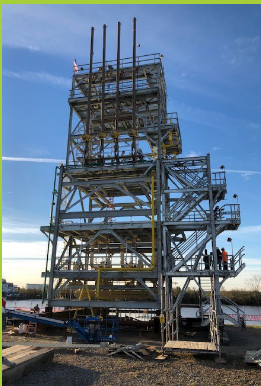
ExxonMobil Dock 5 Retro Fit Project, Port Allen, Louisiana and Baytown, Texas
