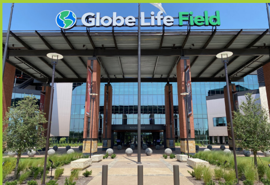
Texas Rangers Ballpark Complex, Arlington, Texas
