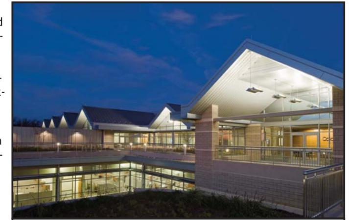
Views at dusk show the complexities and challenges for exterior and architectural lighting. The lower level shows the outline of the perimeter daylight harvest system at night which is raising the light levels closer to full on.
