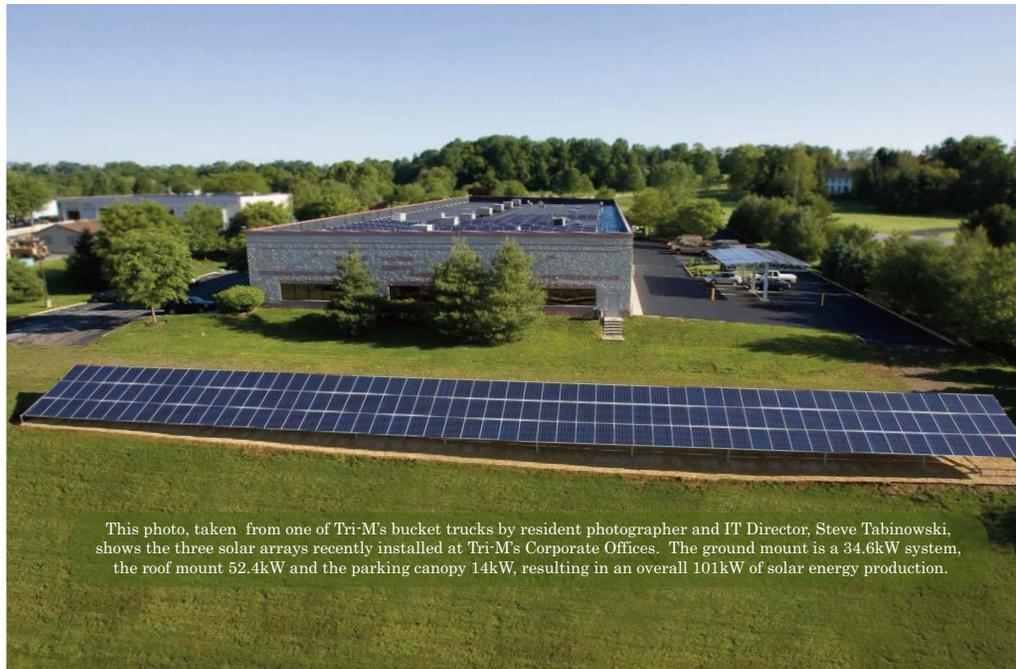
This photo, taken from one of Tri-M's bucket trucks by resident photographer and IT Director, Steve Tabinowski, shows the three solar arrays recently installed at Tri-M's Corporate Offices. The ground mount is a 34.6kW system, the roof mount 52.4kW and the parking canopy 14kW, resulting in an overall 101kW of solar energy production.
